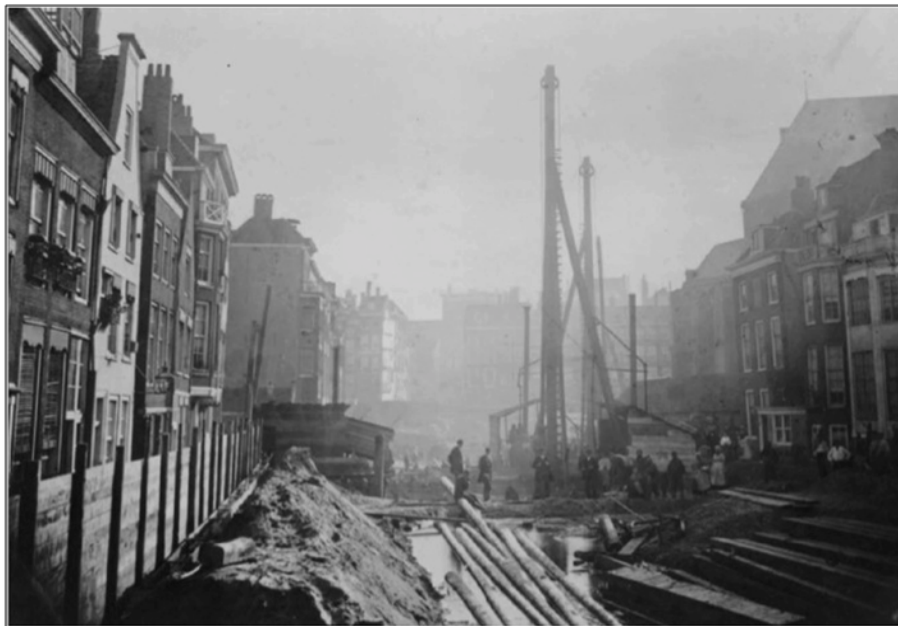
Fig 6.2.3a Centre of Rotterdam. Wooden piles used for the construction of the railroad air track over the trajectory of the former Rotte river. Source: City of Rotterdam
