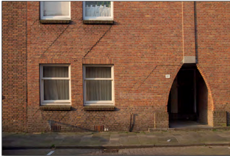
Fig 1.3.1e Various parallel cracks from bottom-right to top-left in wall due to rotting foundation piles. Source: Peter Dorsman
