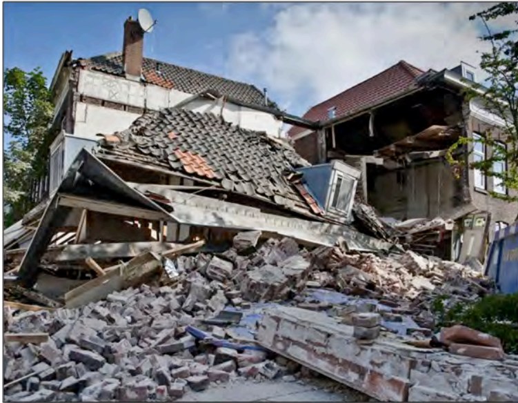
Fig 6.1.10a Drievriendenstraat in the Centre of Rotterdam, June 2013. 19th century houses collapsed due to foundation problems.
